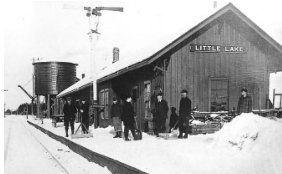
Bahnstation Little Lake
